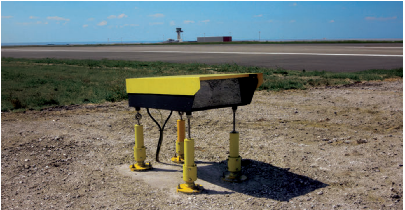
Figure 43: Light unit of a PAPI system at Châlons Vatry aerodrome.
