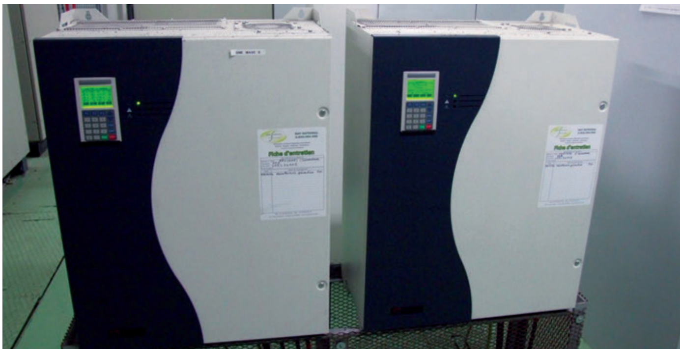
Figure 29: Active harmonic current compensation device SineWave 60 A at Paris CDG aerodrome.
