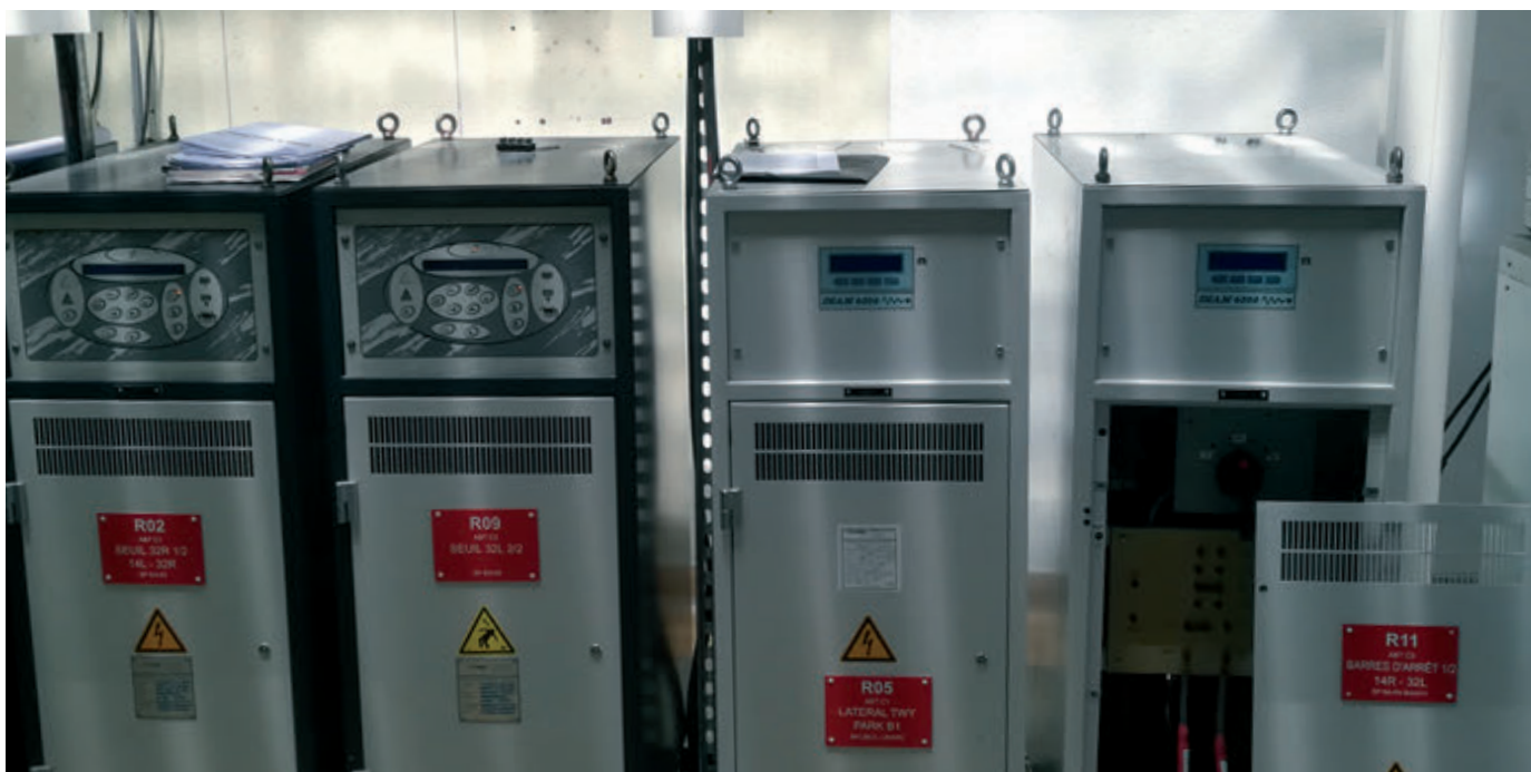
Figure 18: Substation for the power supply of airfield lighting systems at Toulouse Blagnac aerodrome.
