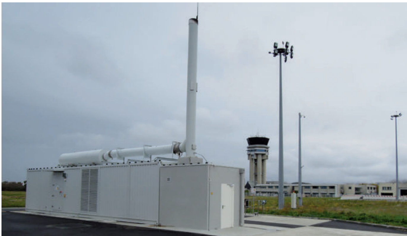
Figure 26: Diesel rotary UPS system in a container unit at Toulouse Blagnac aerodrome.
