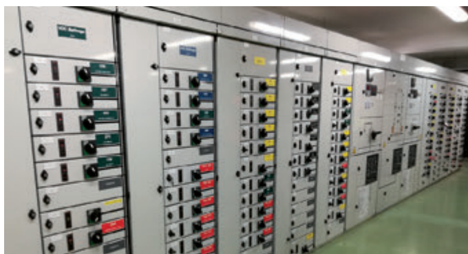
Figure 4: Substation of the power supply system for airfield lighting systems at Paris CDG aerodrome.
