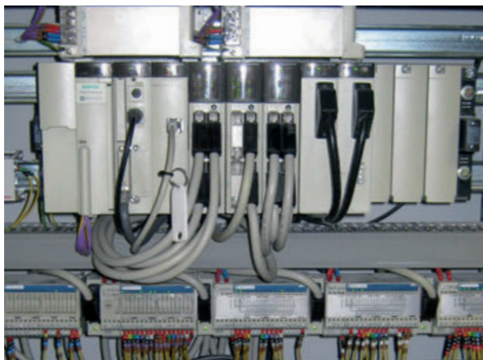
Figure 30: Programmable logic controller at Nice aerodrome.
