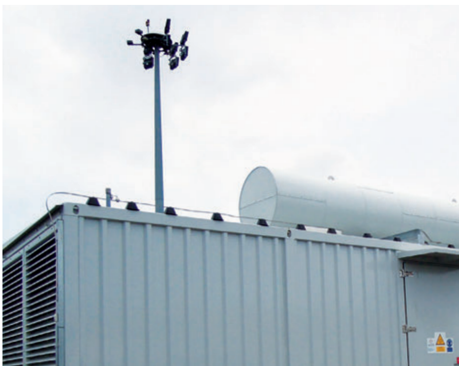
Figure 27: External lightning protection system and lightning air terminal at Toulouse Blagnac aerodrome.
