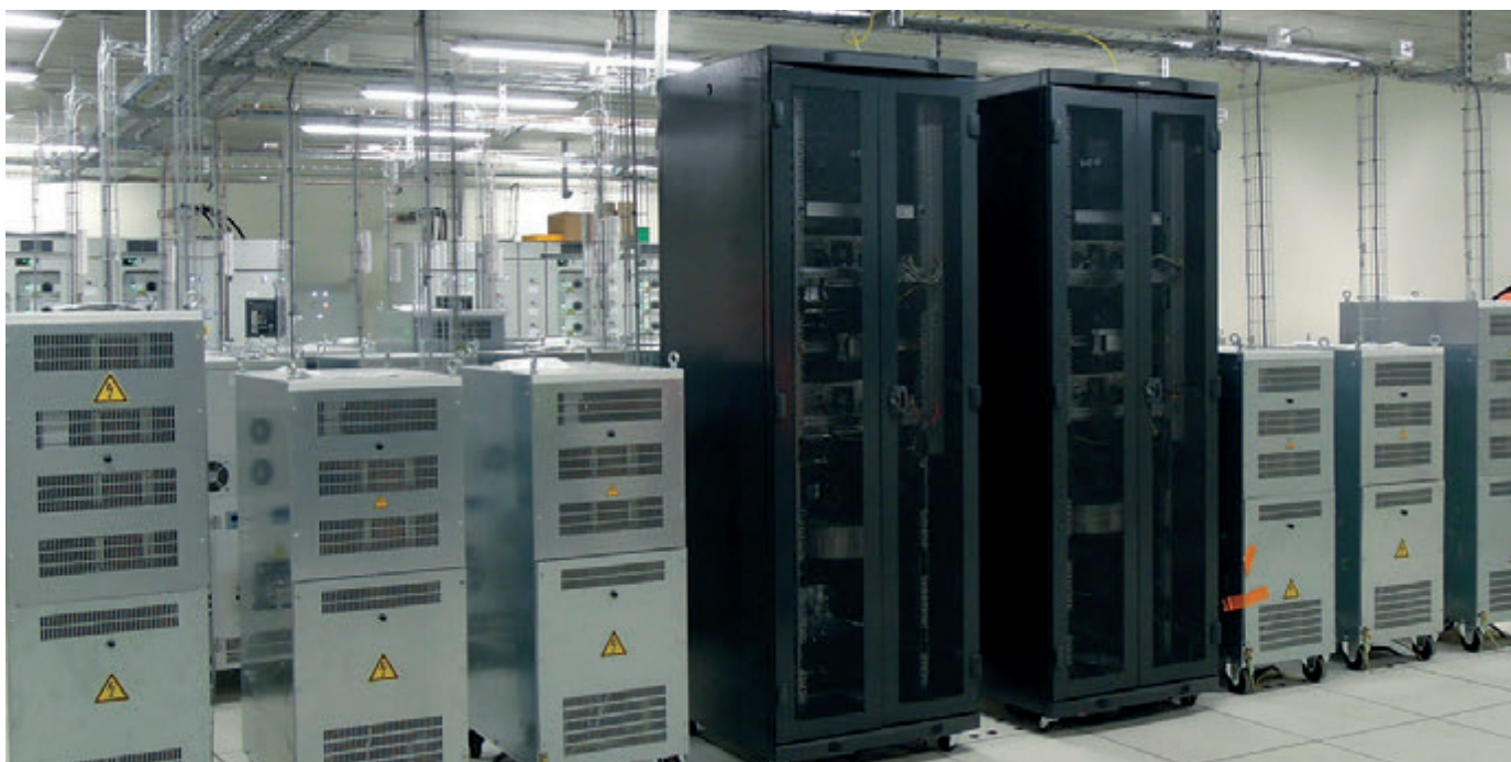
Figure 17: Substation for the power supply of airfield lighting systems at Paris Orly aerodrome.
