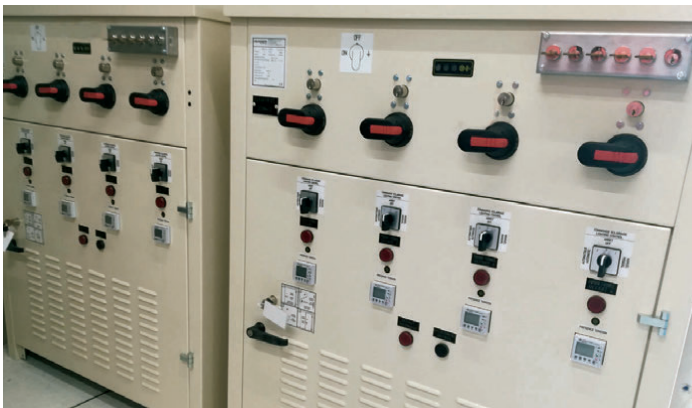
Figure 23: Distribution board for signs and runway guard lights.
