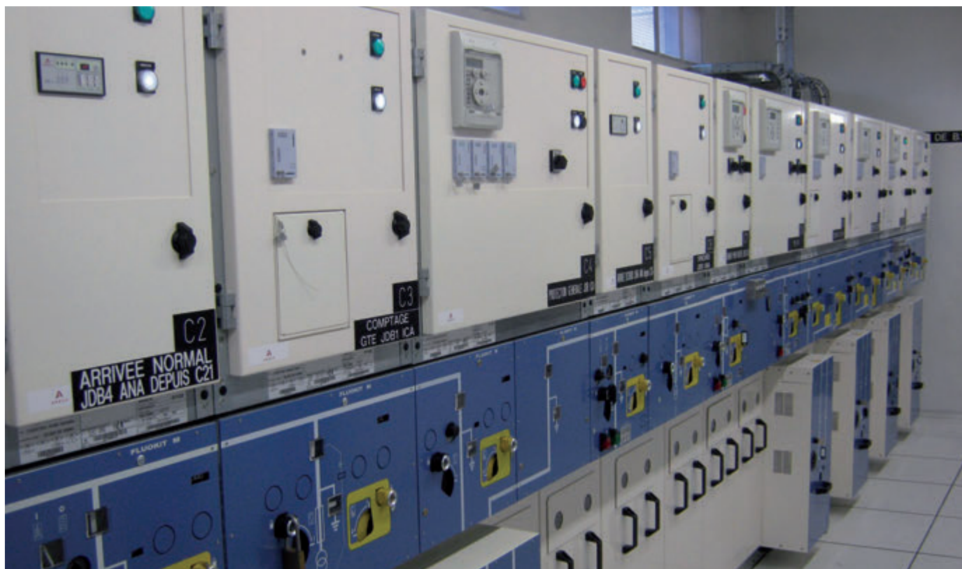
Figure 8: Internal HVA power distribution system at Nice aerodrome.
