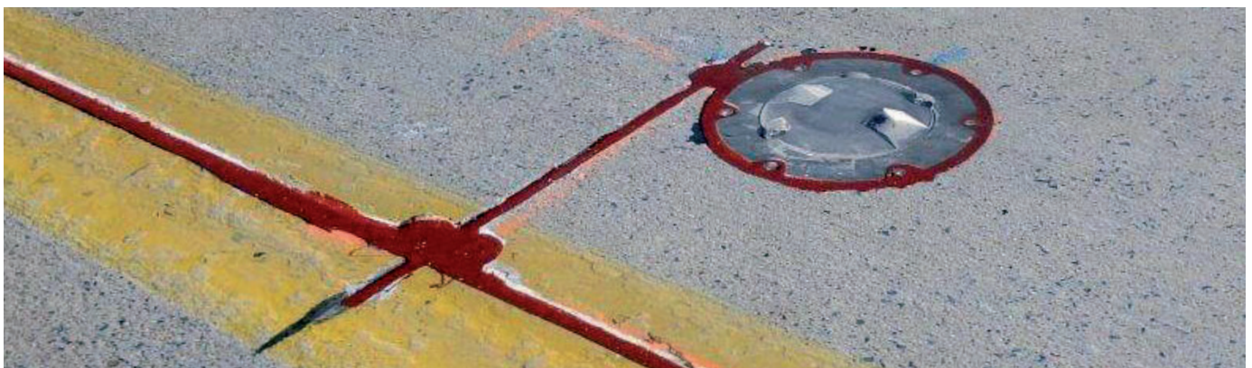
Figure 38: Kerf cut in the concrete pavement of a runway.
