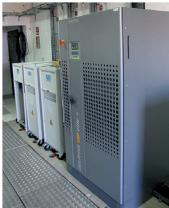
Figure 25: UPS system at Saint Denis La Réunion aerodrome.
