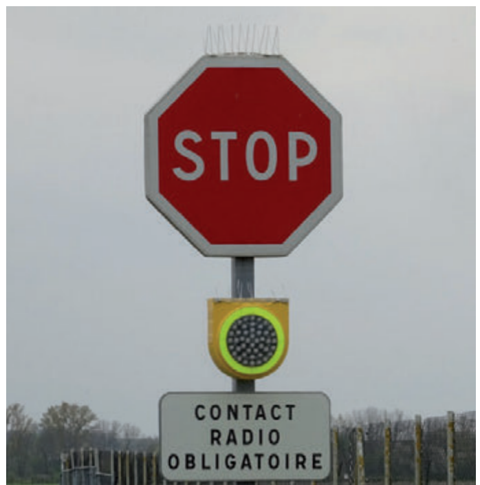
Figure 40: Road-holding position light at Strasbourg Entzheim aerodrome.
