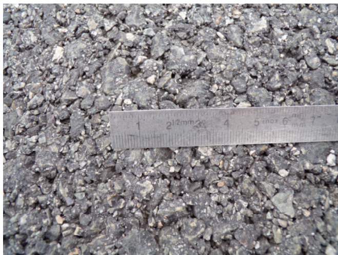
Surface E1: Semi-granular bituminous concrete (0/10)
