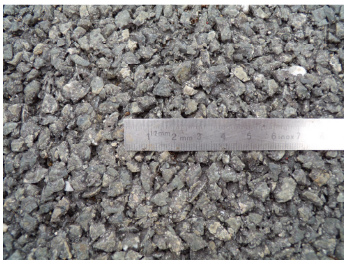
Surface M2: Very thin bituminous concrete (0/6)
