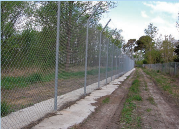
Figure 33 Fence with shutter and burying the fence in concrete.
