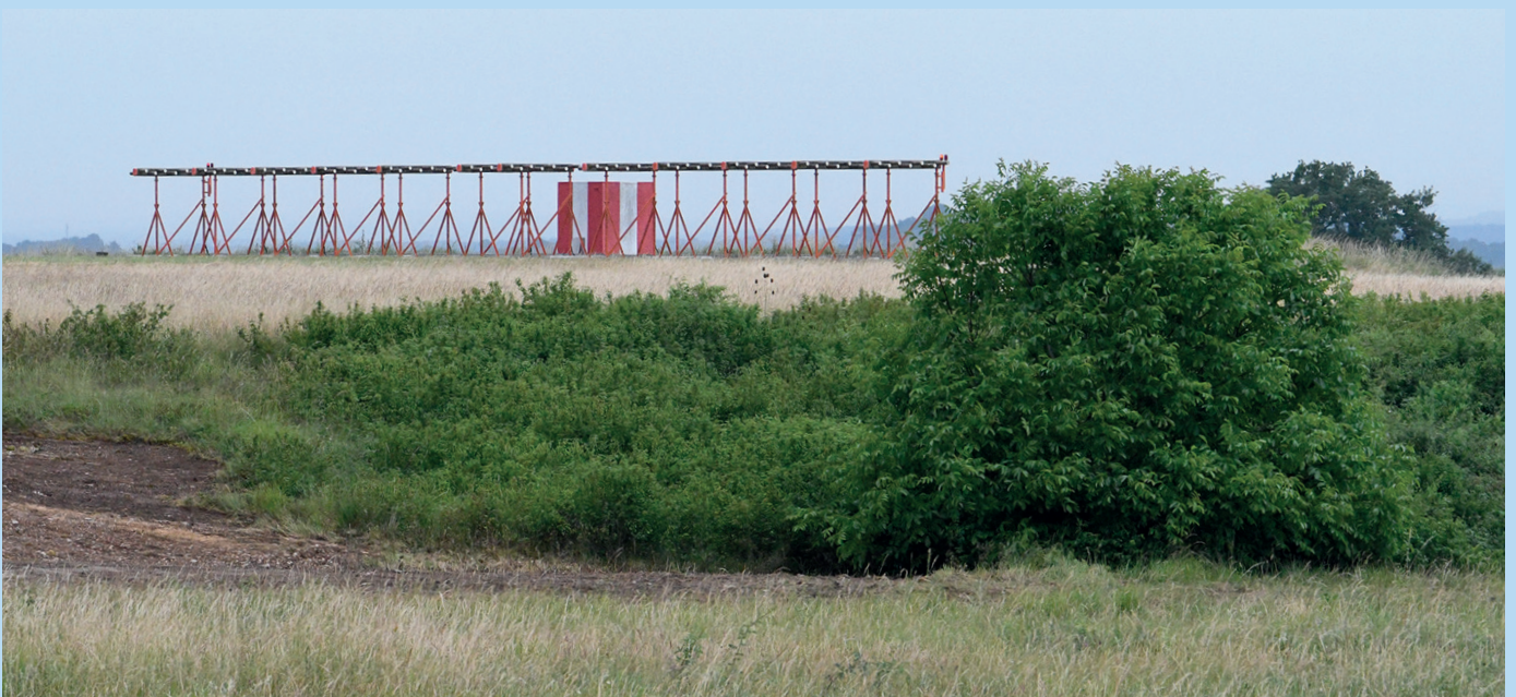
Figure 41 – Refuge area below the runway threshold and localizer at an airport..
