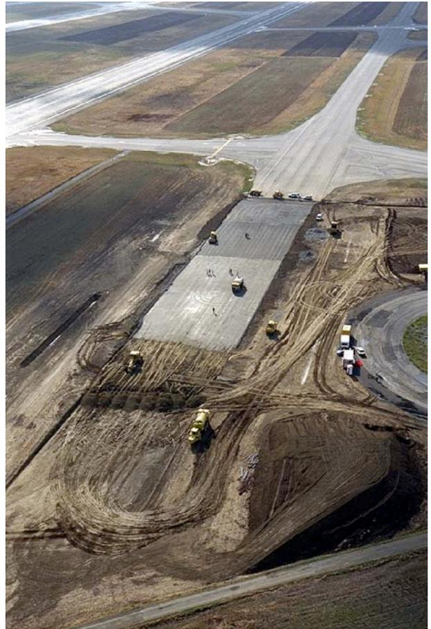
After this phase, a second work stop allowed to set horizontal and vertical strain gauges in the GRH course and at the base of the base course (see a forward section).
