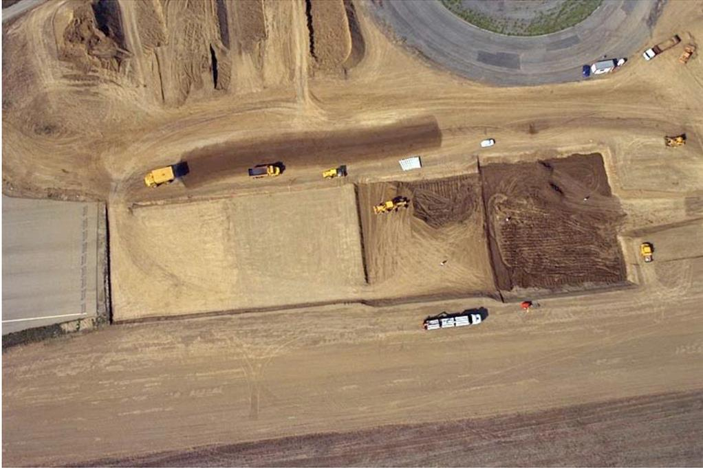
Continuous EV2 tests allowed to build homogeneous layer: for example, when theoretical water susceptibility was too low, resistance to deformation (measured by EV2 test) was too high, the subgrade was scraped and sprayed with water until obtaining the specified values. Inversely, the subgrade was scraped when weather was sunny to dry the subgrade.
