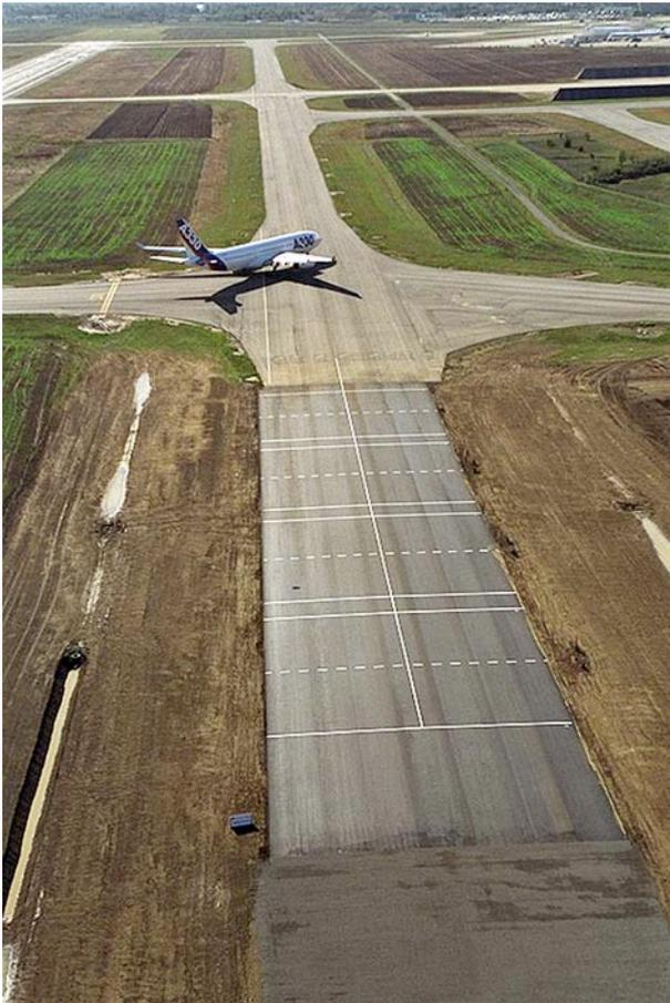
These courses were used by two teams each constituted by one finisher, one pneumatic tire roller and one compactor, for two reasons: quality (hot longitudinal joint, best compaction) and full capacity.
