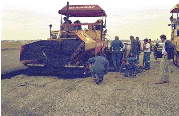
The sensors placed at the base of the bituminous layer were glued on the surface and covered by some asphalt taken from the feed hopper of the finisher. Then they were foot-compacted before the finisher was allowed through. Precautions were taken, in order to prevent the finisher from running over the sensors. Roller was used without vibration for smoothing during surface finishing.
