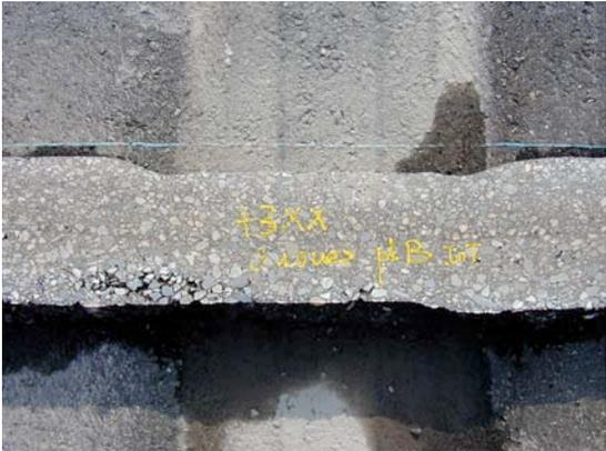
**Example of a trench wall-side located on structure B, in the A380 bogie 6-wheel-path**
